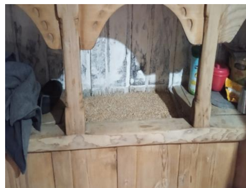
Fig 4: Kothar built inside the home for storage of cereals
