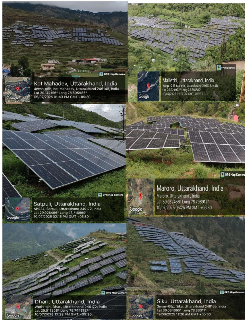
Fig 4. Showing the ground mounted SPP in the study area (Collected during field survey)
