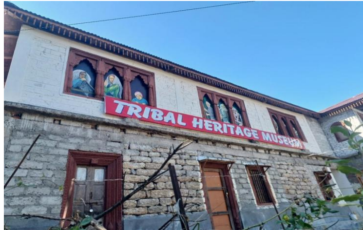
Fig 7: Tribal Heritage Museum at Munsyari, Pithoragarh (Uttarakhand) Source: Photo taken by the author
