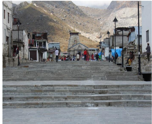
Fig.1: Street widening & grading
